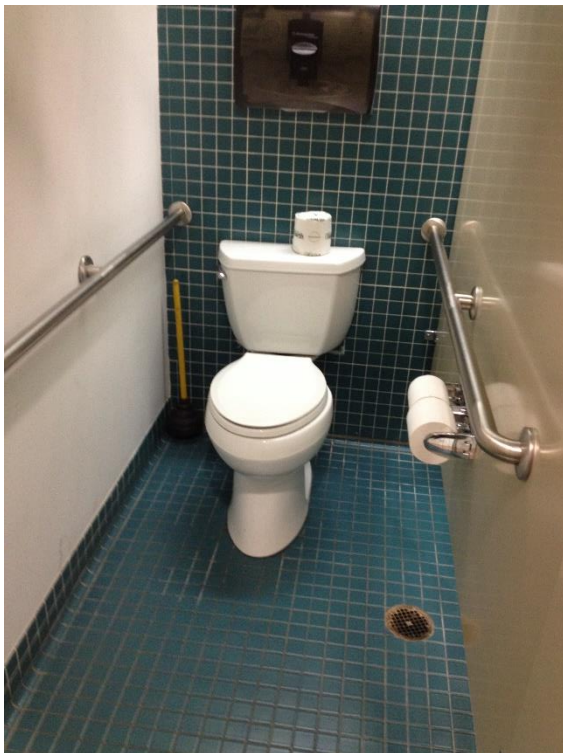
Toilet stall does not comply with current ADA
