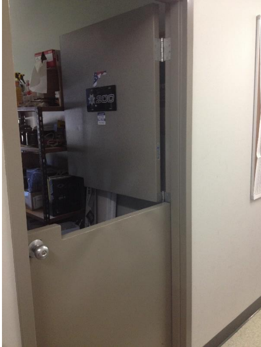
Fire door must be on closers or hold-opens to release in the event of a fire. Charging stations for radios and flashlights in makeshift location.
