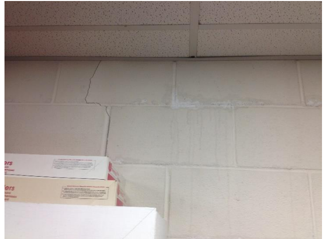
Cracks in wall at break room and stairwell.
