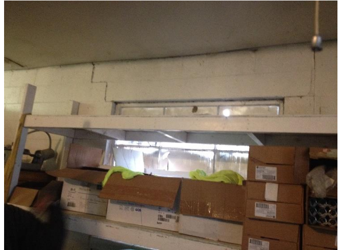
Structural Cracks to be addressed
