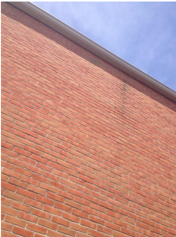
Stain on exterior indicates likely location of water infiltration In south wall at Parapet.
