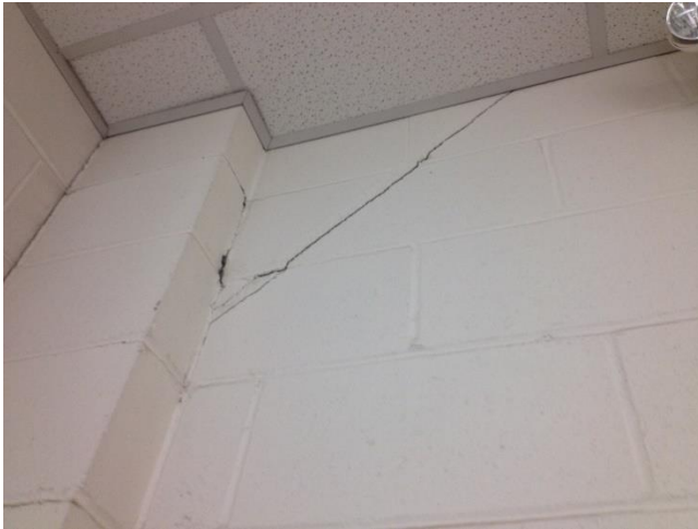
Cracks in wall at break room and stairwell.
