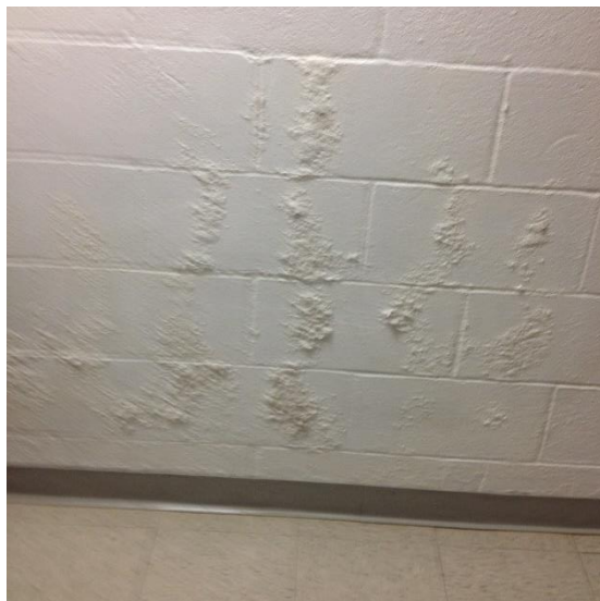
Evidence of moisture infiltration in basement walls
