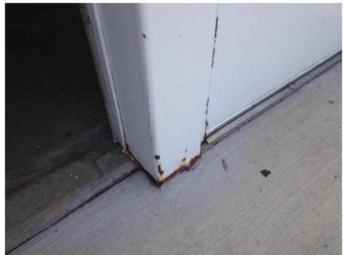
Heaved stoop at exit door causes door to bind
